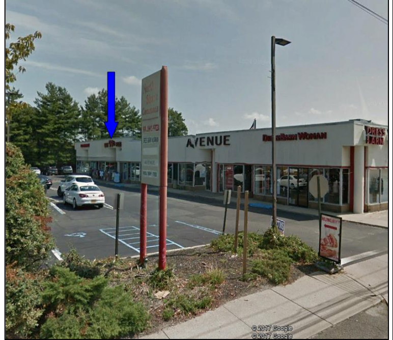
STREET VIEW (LAKEVILLE RD)
