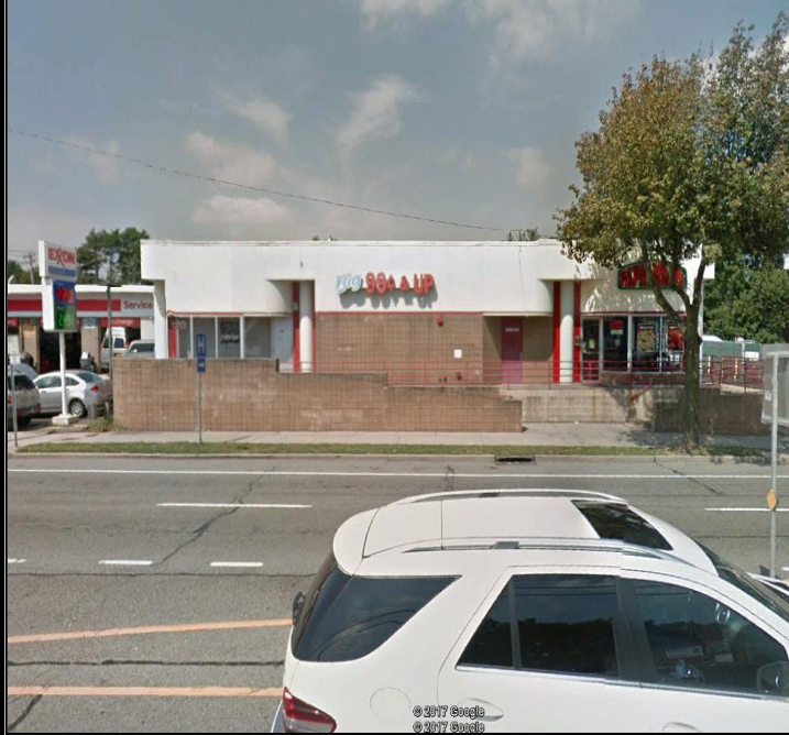
STREET VIEW (HILLSIDE AVE)
